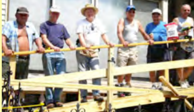
Central Berks Lions install new ramp at the Kunkel's home
